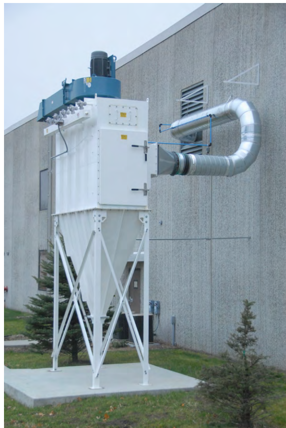
Arrangement 4VI (vertical, inlet mounted) on baghouse dust collector.
