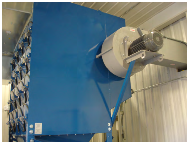
Arrangement 4HI (horizontal, inlet mounted) on a cartridge-style dust collector (support by customer).
